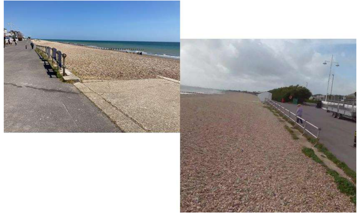
Figure 22 - Nyewood Lane, May 2023 and Sept 2019
