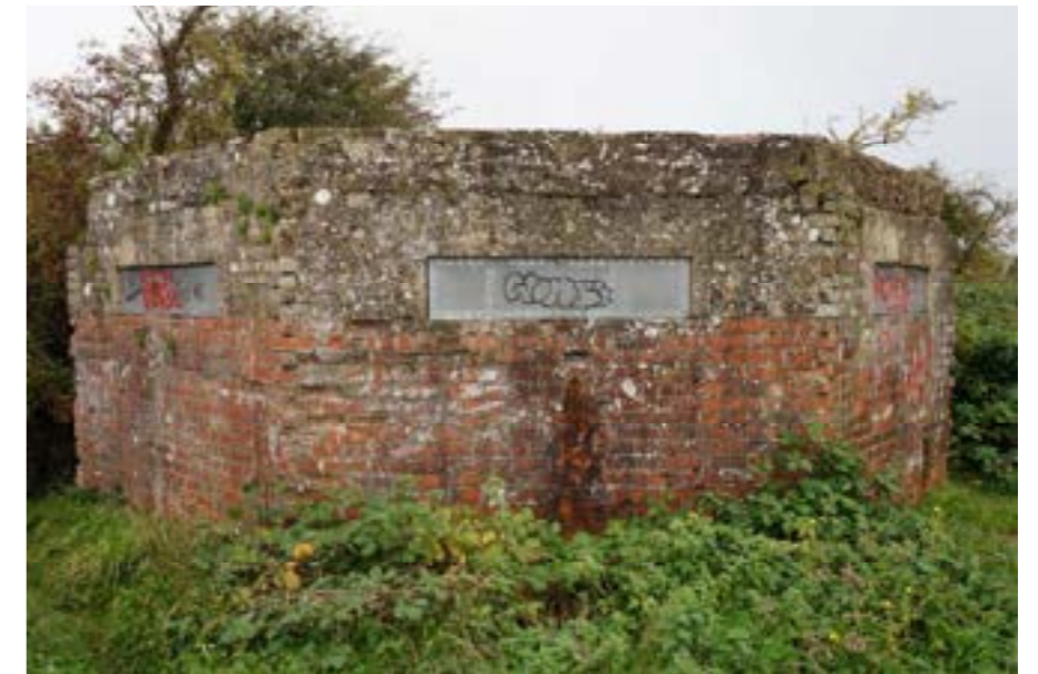
Photograph 8: Pillbox within Western Field
